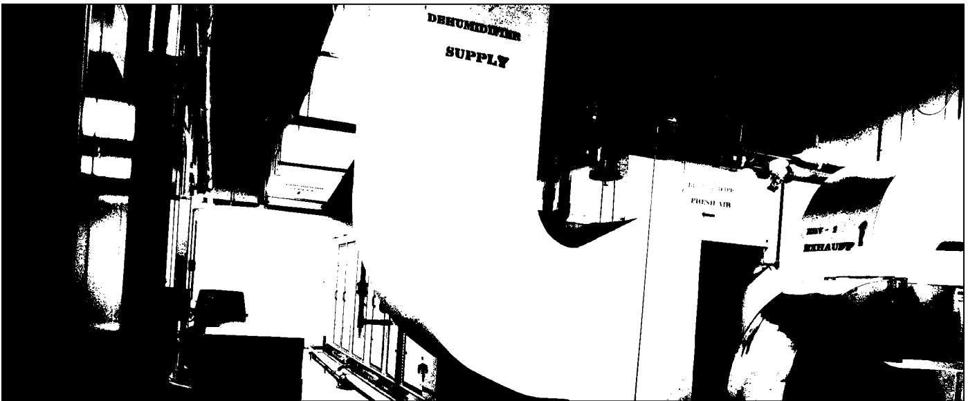
Pool area HVAC mechanical room at the Central Labrador YMCA
