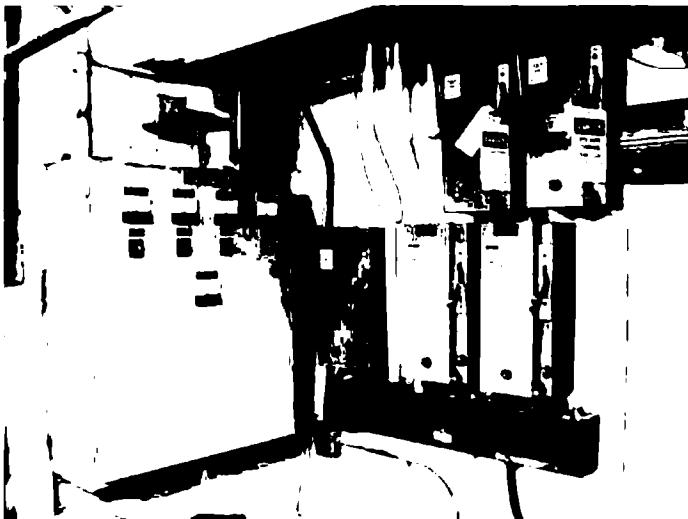
Pool Pump Room - Abandoned South Wall Equipment
