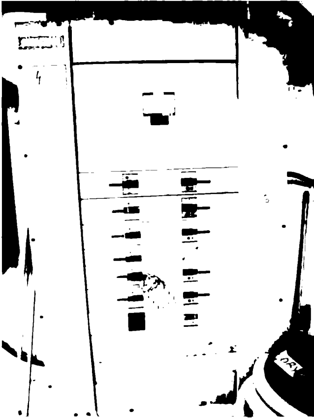
Pool Pump Room - Distribution panel for pool heaters, pumps and controllers.
