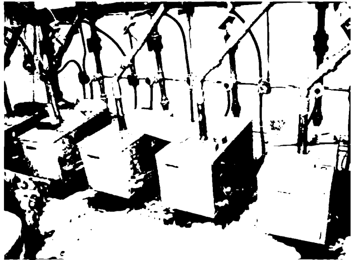
Pool Pump Room - Electric pool heaters.
