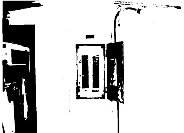
Work Shed - Breaker panel.
