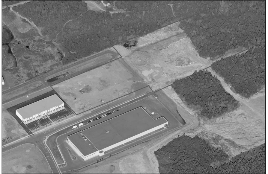
Aerial View of Subject Property Showing Approximate Boundaries
